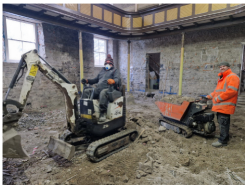
Work progressed on excavations for the new, insulated ground floor
