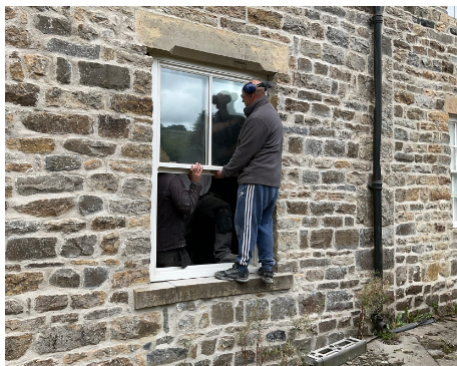
The first element of the restoration was the replacement of the windows in the north and south elevations with new double-glazed, sliding sash units
