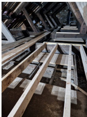
A new access hatch into the roof void was formed to enable repairs to the roof structure to be completed and safe maintenance platforms installed
