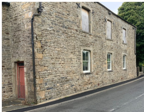
The first element of the restoration was the replacement of the windows in the north and south elevations with new double-glazed, sliding sash units
