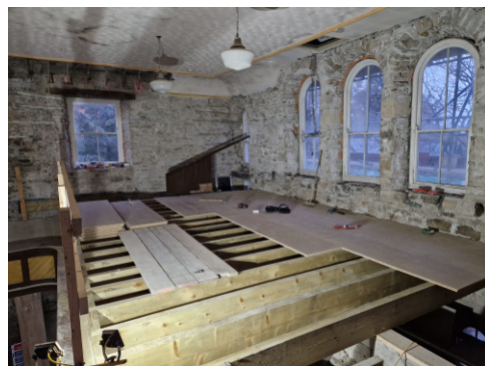
and on the new, timber first floor structure to provide a large area of levelled gallery.
